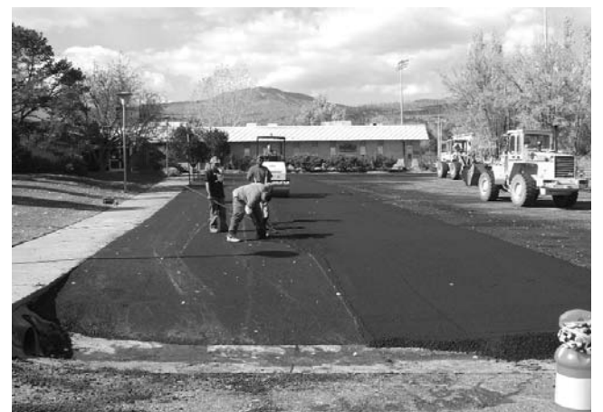
Repaving the parking lot.
